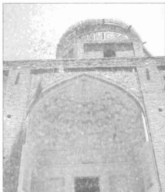
15. Moshâtâqiyeh (Kowsar iwan and dome)
